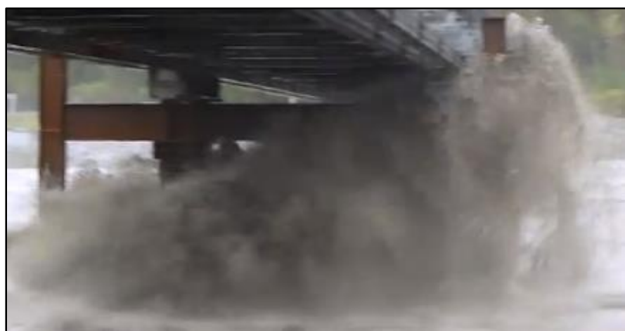
Figure 5-2 – View showing resistance at Waiho Bridge Pier during flood event
