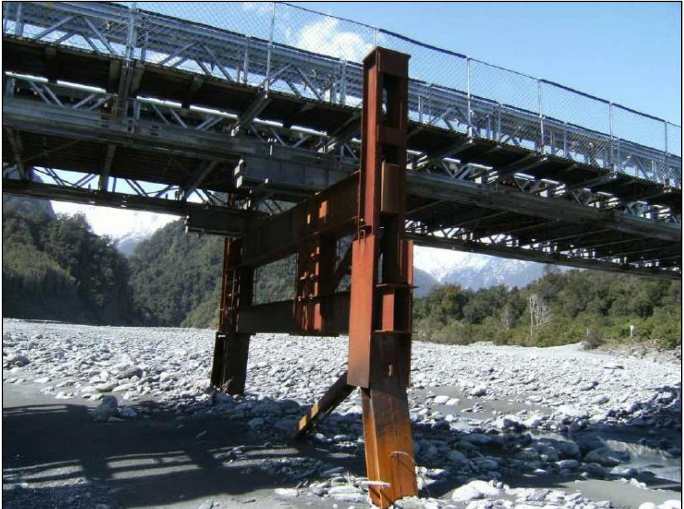
Figure 4-2 - Photo of a typical bridge pier (Opus, 2011)
