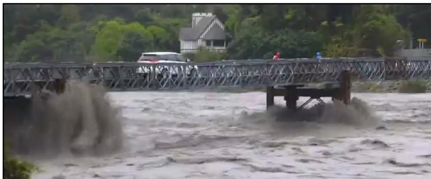
Figure 5 -1 - View of Waiho Bridge in flood (view looking downstream)
