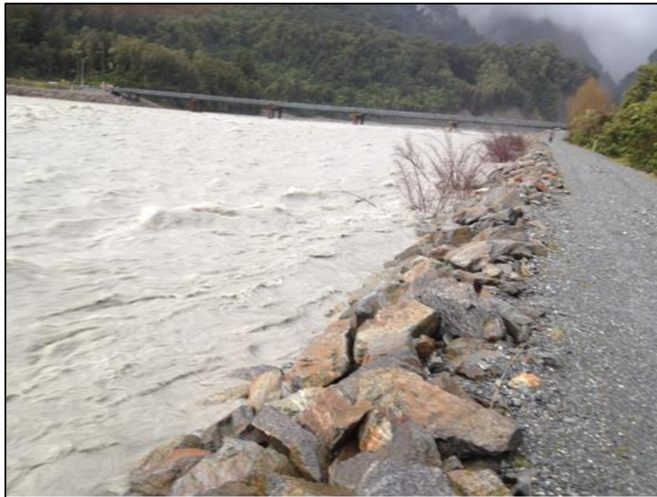
Figure 5-4 – Water level adjacent to motel units on the 23rd May 2014
